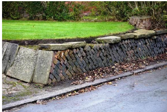
Boundary treatments along Church Lane
