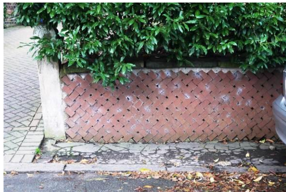
Boundary treatments along Church Lane
