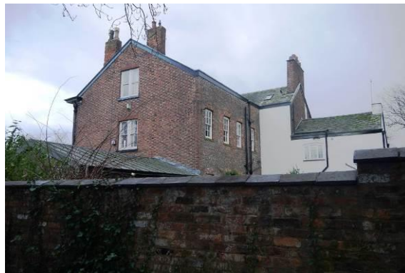
The rear of Ashton New Hall
