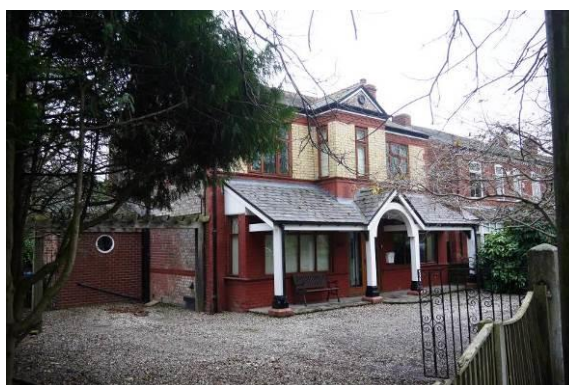
Mid-20 th century addition to the Conservation Area
