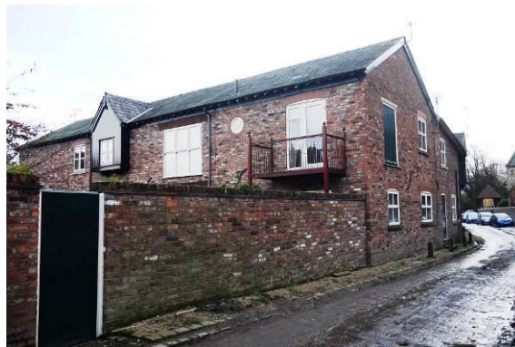
The rebuilt north end of the Mill development
