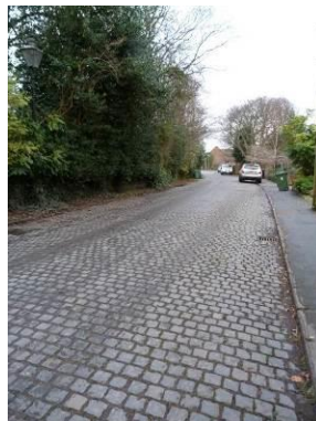
Road surfacing within the character zone
