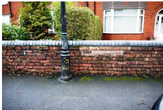
Boundary treatments along Church Lane
