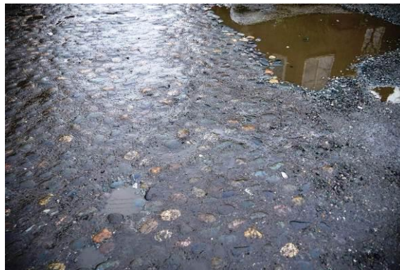
Paving east of Church Lane in front of the farm
