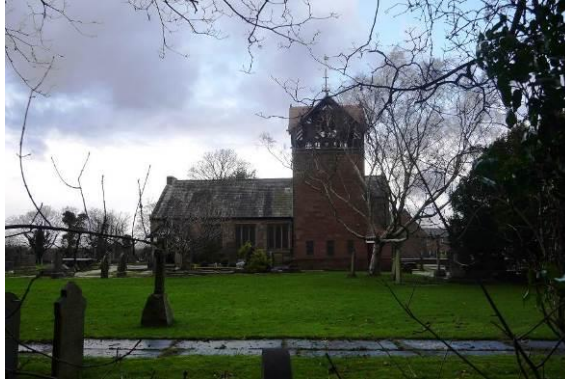
View of the church, south elevation
