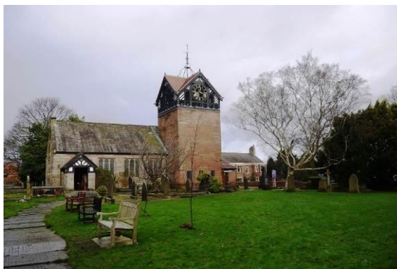
View of the church, south elevation
